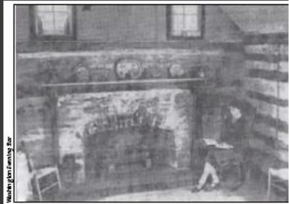
Mrs. Bolten in Log Kitchen after renovation in 1939
